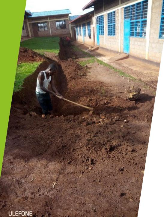
Water trapment using Swales
