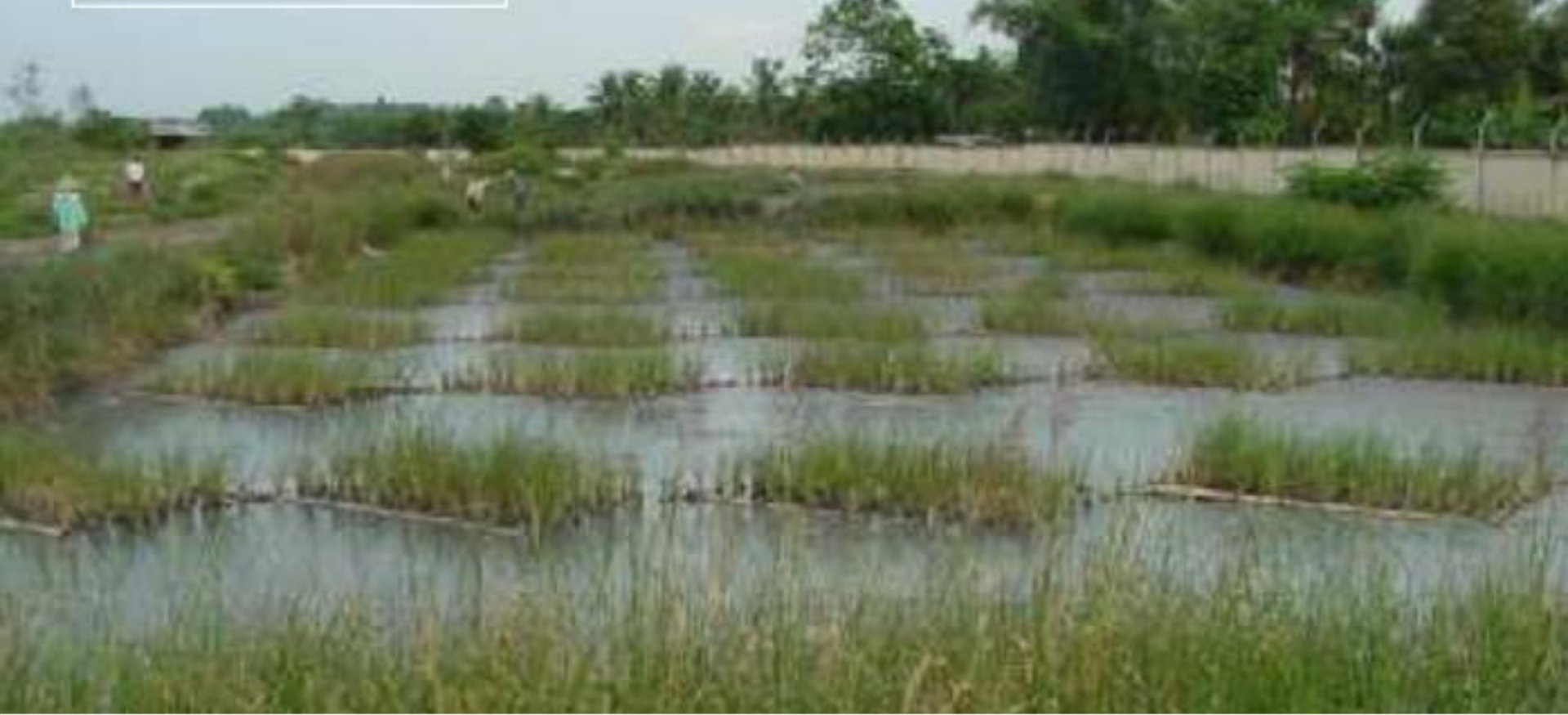
Water treatment in Vietnam
